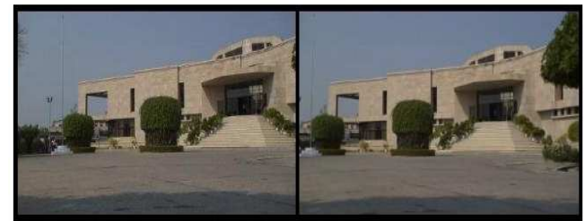
Fig.6 Images taken by the robot while facing the building in the outside environment
